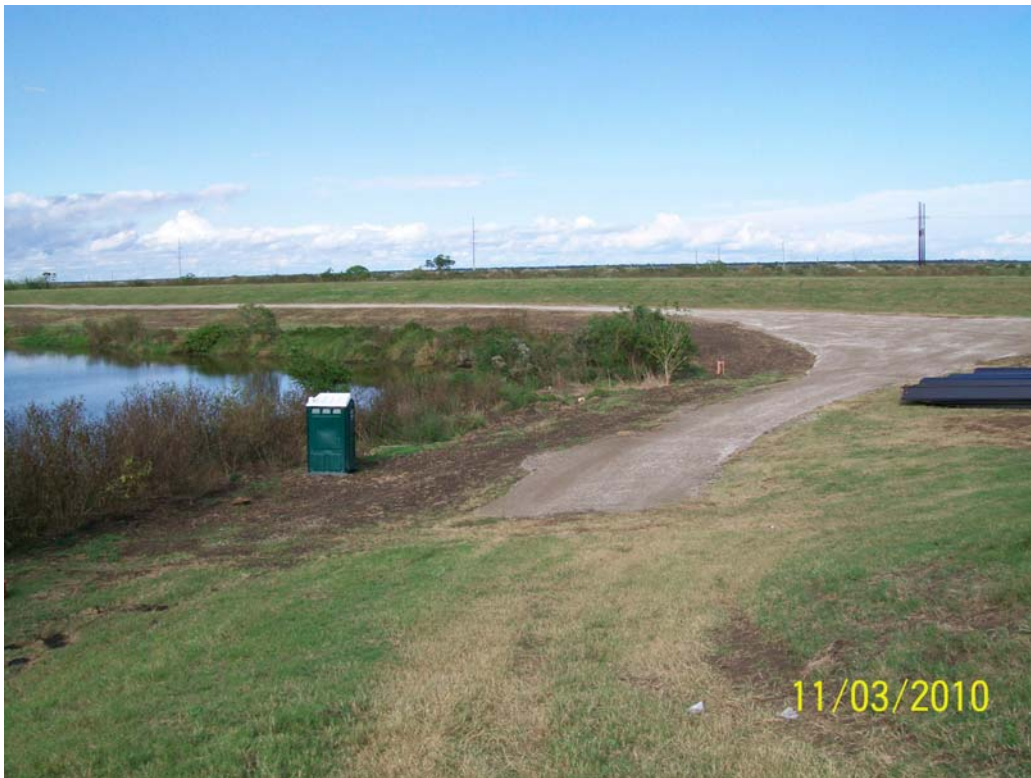
Violet Canal Structure construction access road near to closure structure
